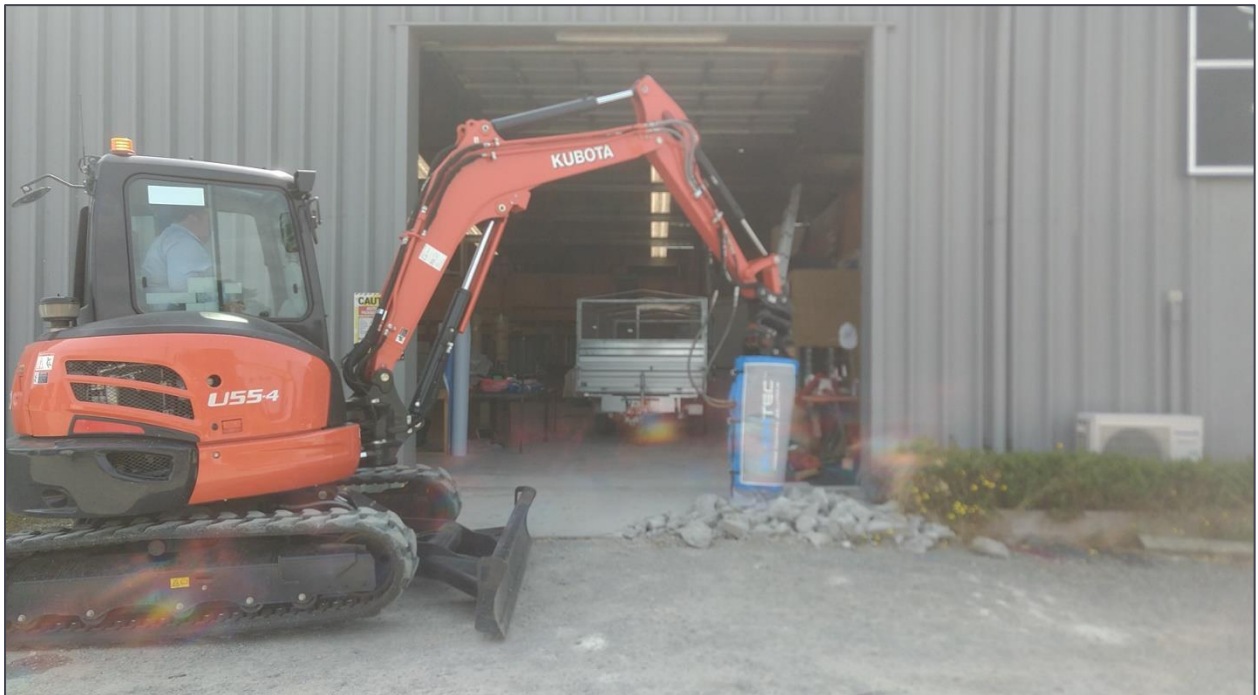
Figure A1: With rock breaker attachment
